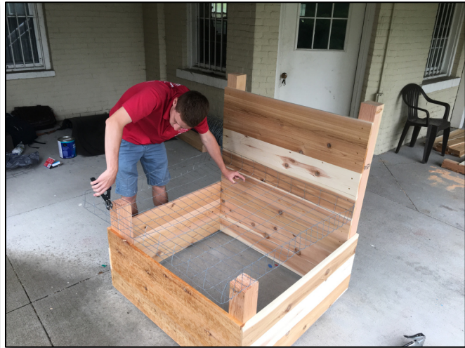
2. Cut out corner sections of fencing to create flaps, and to make space for corner posts
