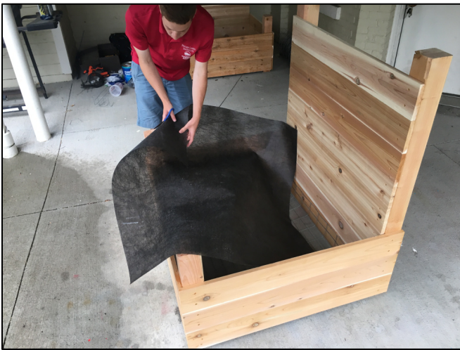
3. Fold 8' x 4' sheet in half to make a 4' x 4' sheet, cut corners for flaps, and staple on top of wire fence
